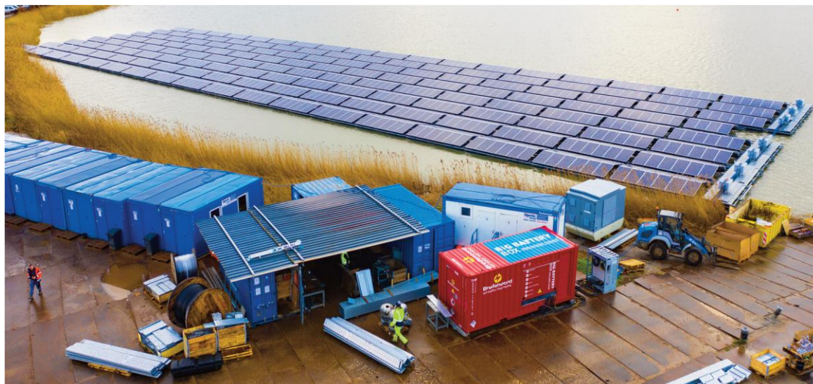
Sekdoorn FPV Park, Netherlands
