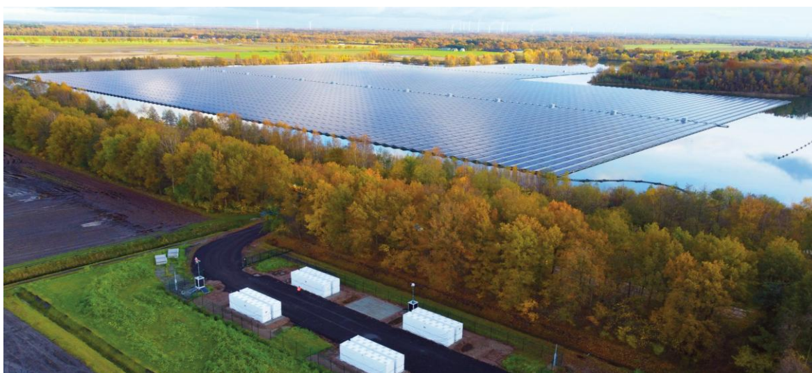
Sellingen Floating Solar PV Park with battery storage Netherlands
