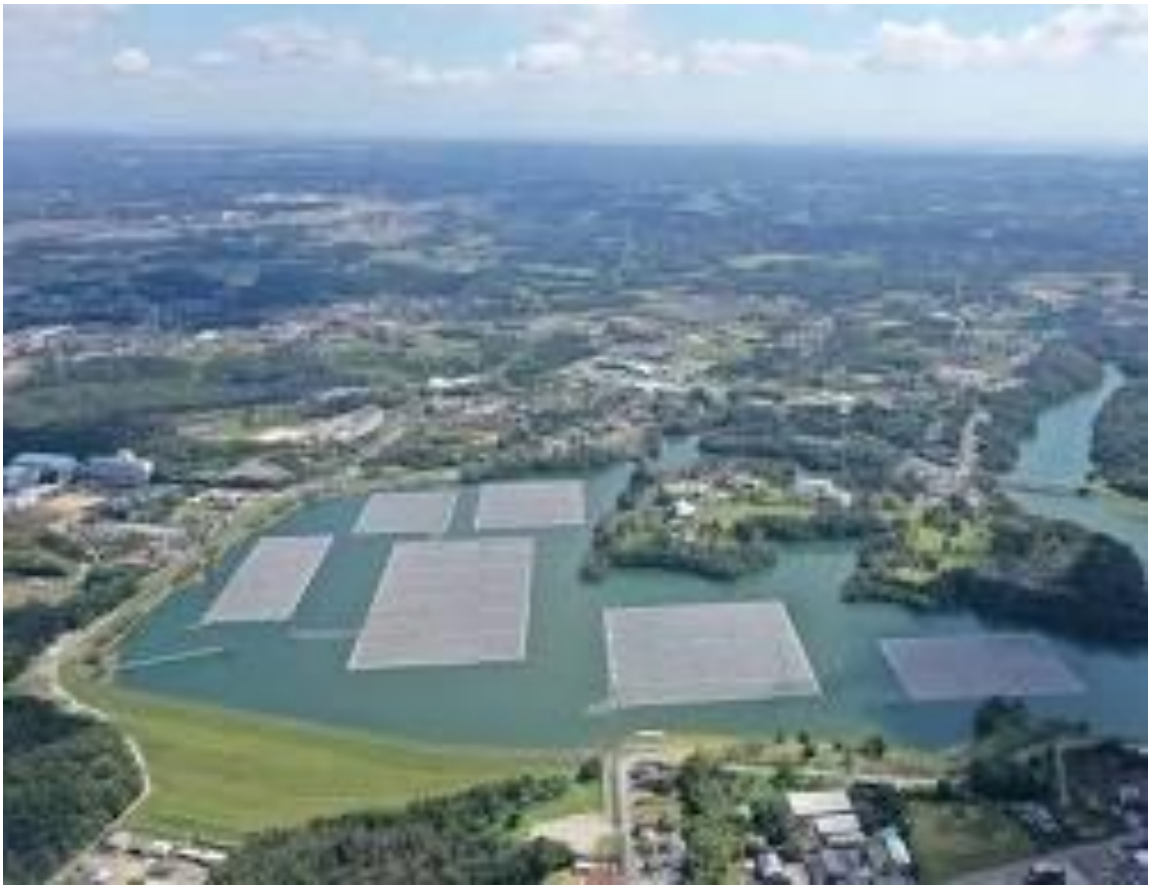
Yamakura Dam Floating Solar Plant, Japan
