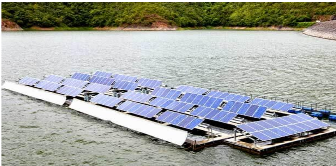
Mudasarlova Reservoir Floating Solar Power Plant, India
