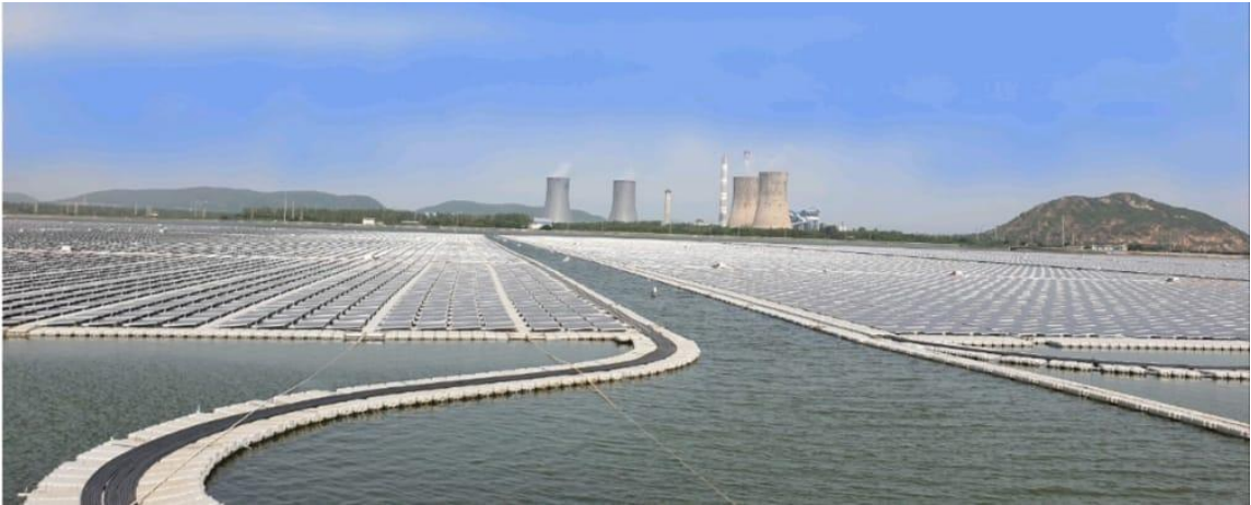
Simhadri Floating Solar Power Project, India
