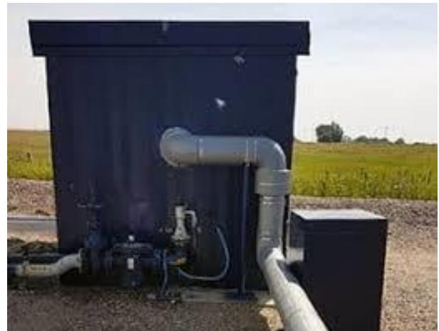
*Figure 45: Insulated pressure vessel and pipe*
