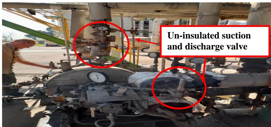
*Figure 29: Uninsulated portions of Turbine Pump*
