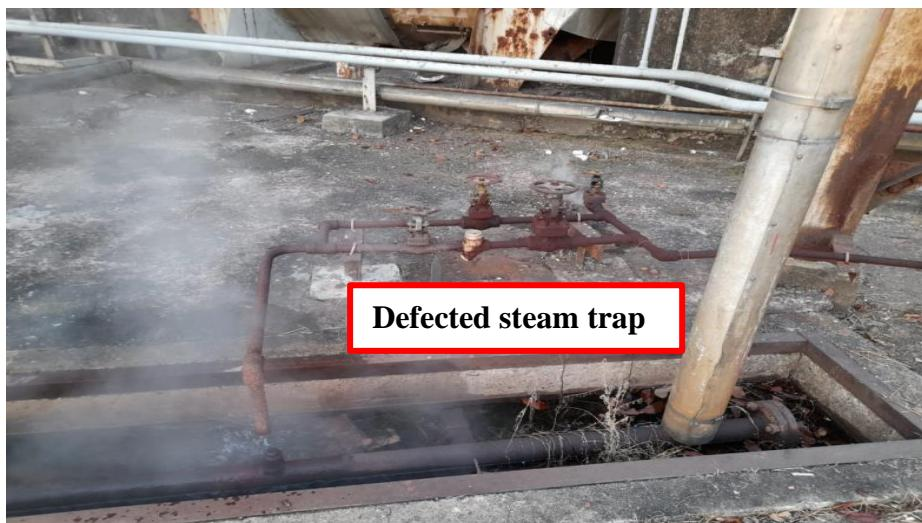
*Figure 27: Defected steam trap*
