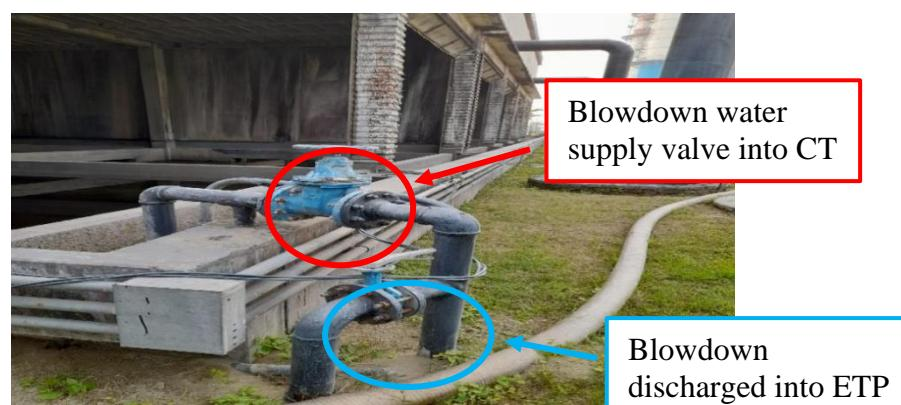
Figure 25: Usage of blow down water as cooling tower makeup water.
