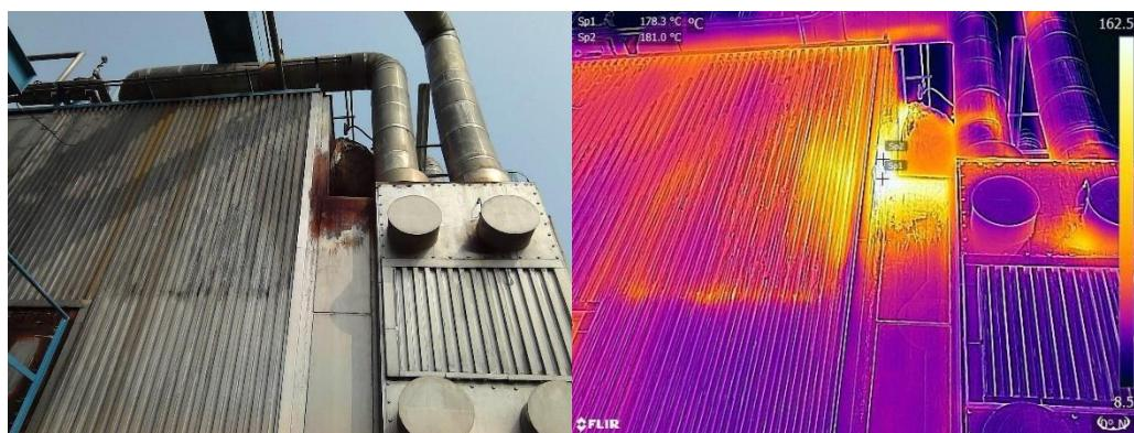
**Figure 16: Hot spots of the auxiliary boilers**
