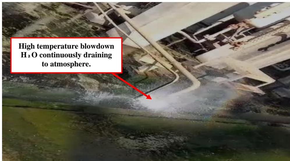
*Figure 33: Heat Loss with blowdown water*
