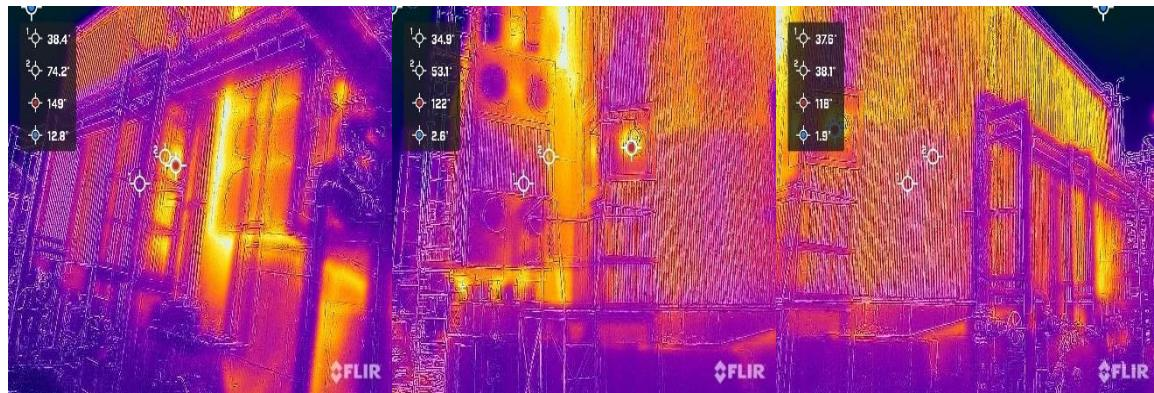
**Figure 12: Good thermal insulation of the other surfaces of the auxiliary boilers**
