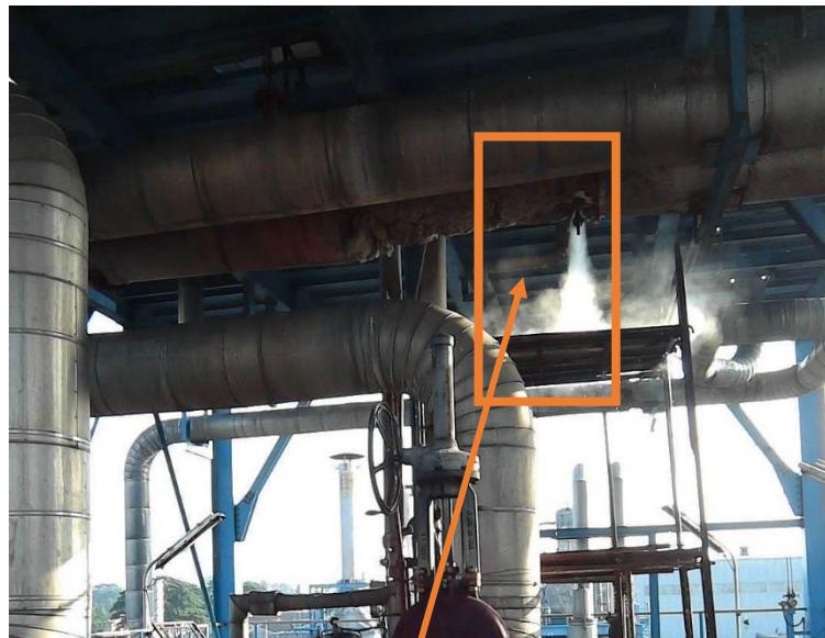
**Figure 10: Steam leakages****Table 12: Energy savings by repairing steam leakages**
