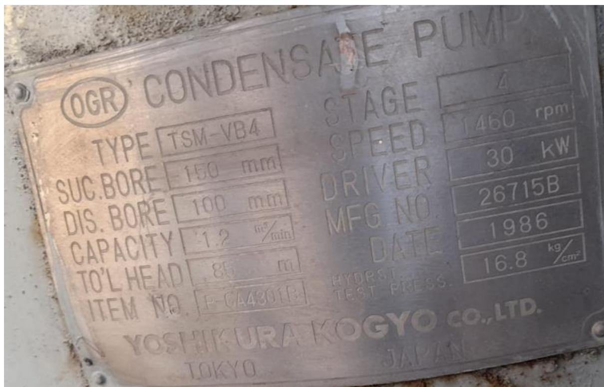
Figure: Condensate Pump technical datasheet.
