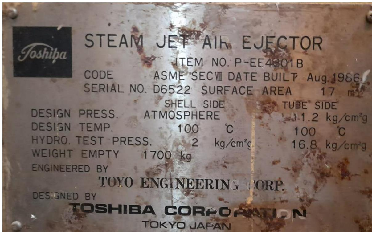
Figure: Steam turbine ejector technical datasheet.
