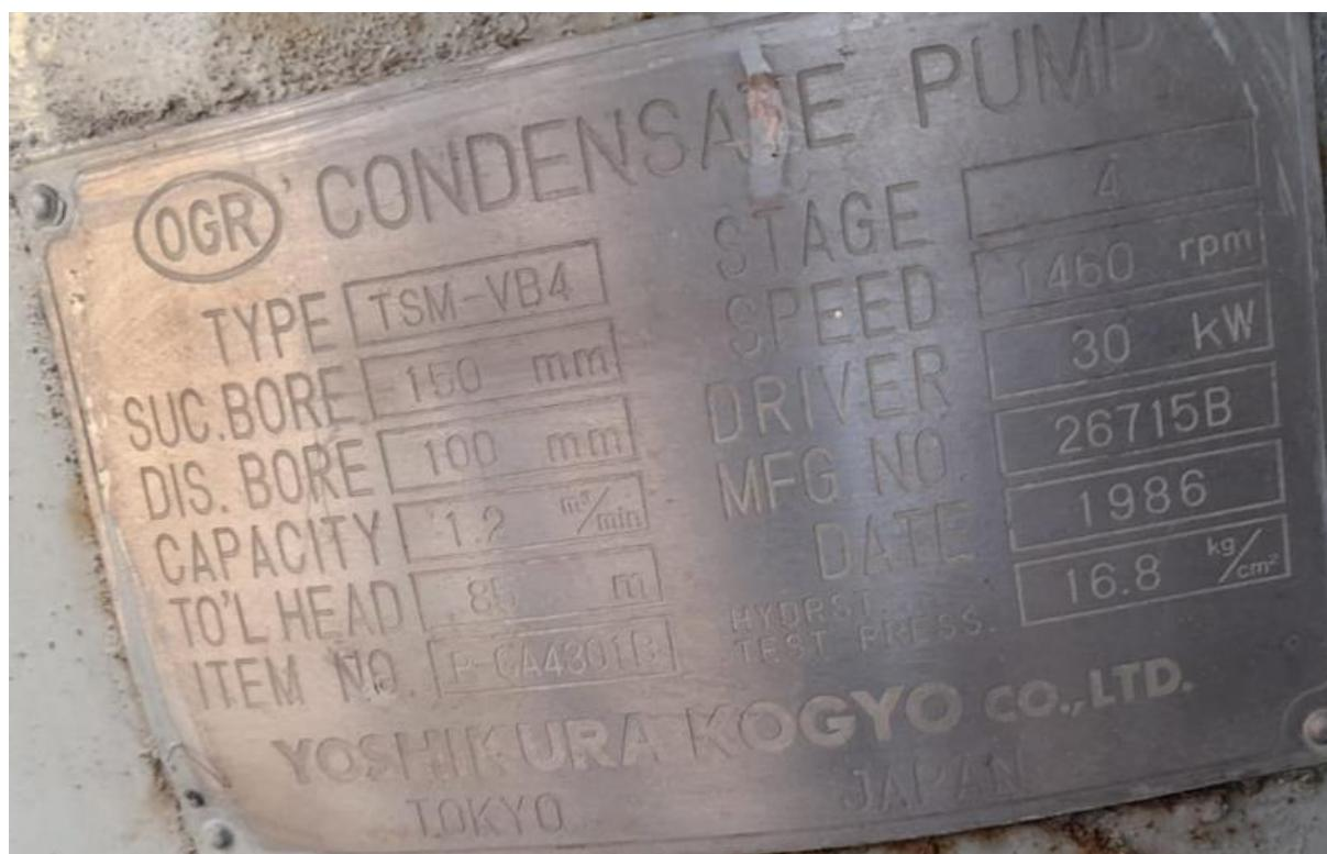
Figure: Condensate Pump technical datasheet.
