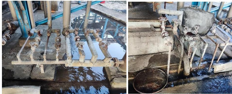
**Figure9: Steam traps****Table 11: Energy savings by repairing steam traps**
