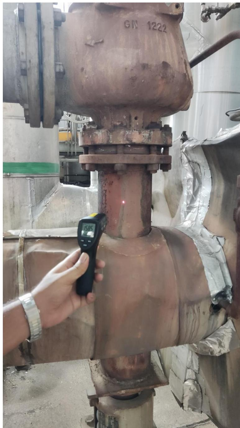
*Figure 2.7.1: Uninsulated Portions of Turbine Pump*
